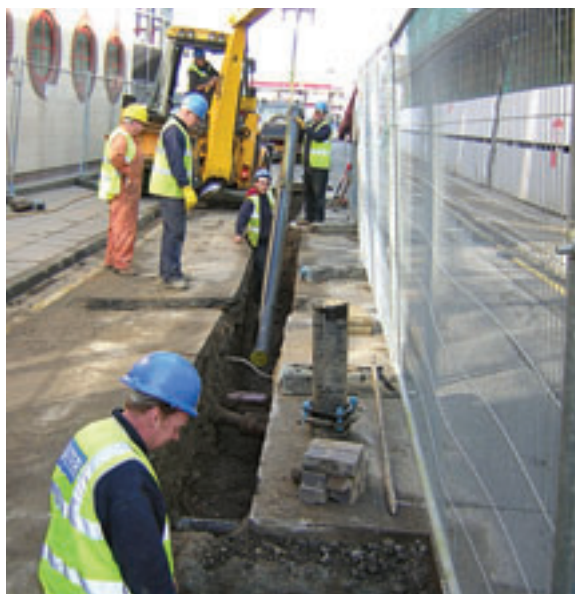
Laying of a replacement 150mm diameter water main in St Helier
