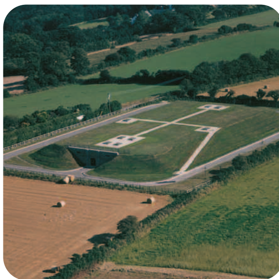
Les Platons treated water service reservoir
