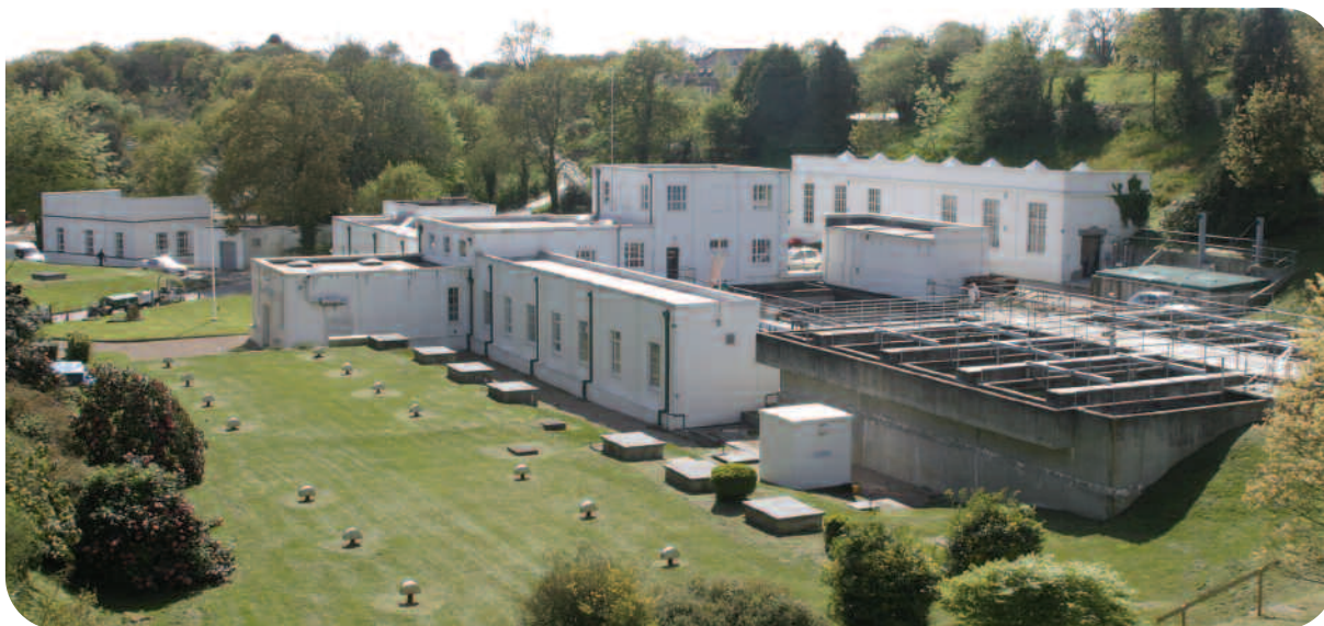
Handois Water Treatment Works
