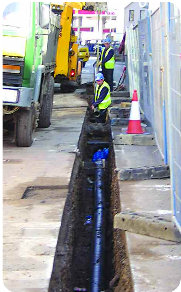
Foreman Kevin Bassett and Joe McGowan laying a replacement 150mm diameter water main in St Helier
