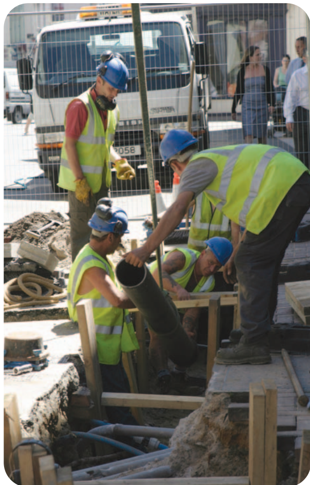
Work undertaken in Union Street
