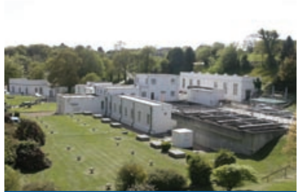
Handois Treatment Works
