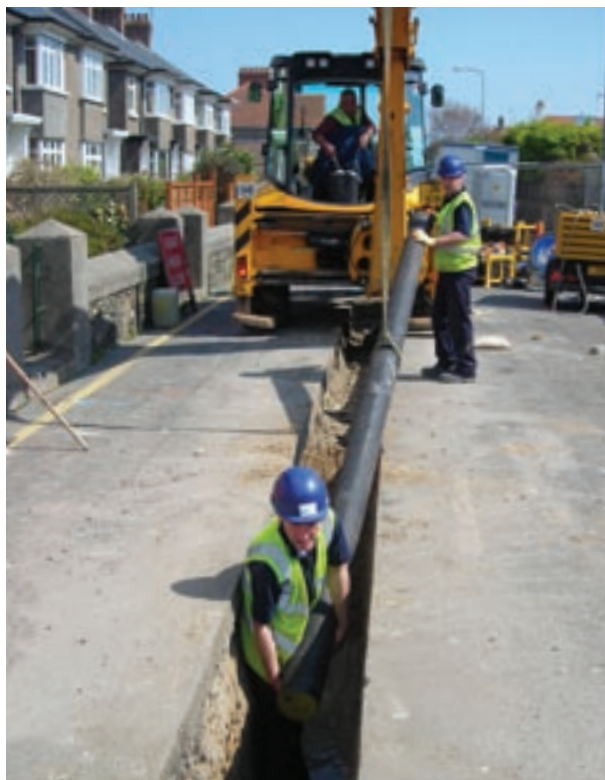
Mains renewal in Green Road, St Clement.
